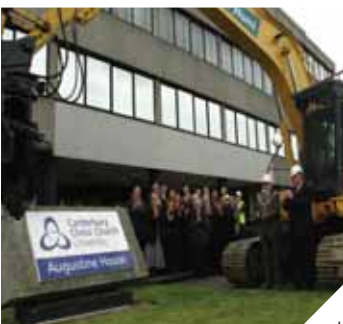
Demolition began at the site of the new Augustine House in November
