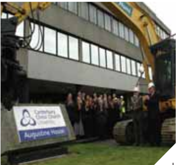
Demolition began at the site of the new Augustine House in November
